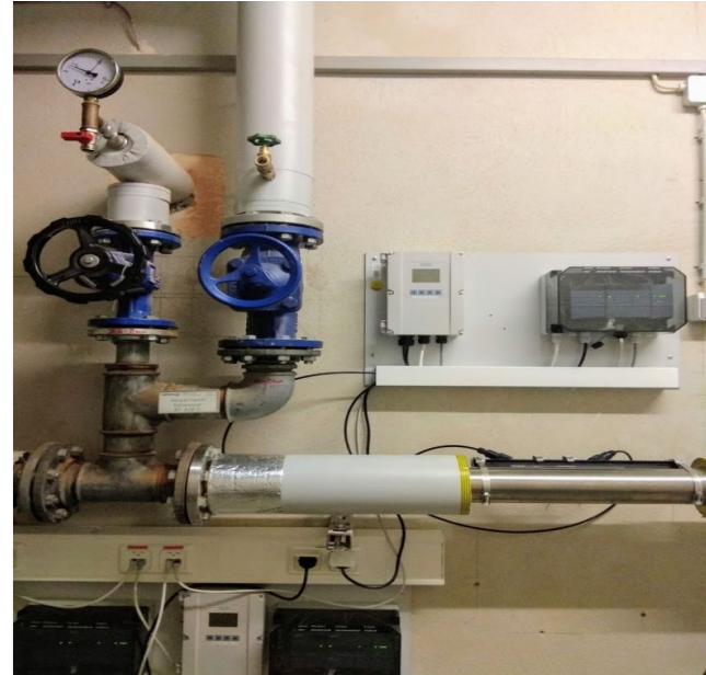
Hardware setup for the acquisition of water data at the UAS Landshut.
